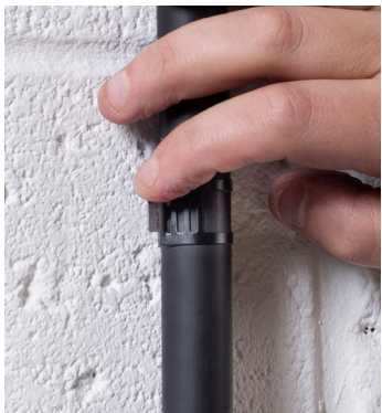
Select notch according to cable dia & secure with locking tab
