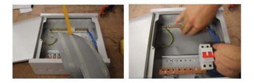
4) Should there be a large number of cables to come through the back of the unit and fitted to a hollow wall, a sleeve can be fitted in place of the back gasket Made in two sizes but easily cut down to suit other size holes
