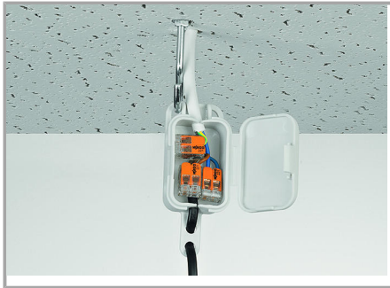
Pendant light connection in suspended ceilings
