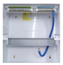
Disconnect Blue Cable and remove Main Switch
