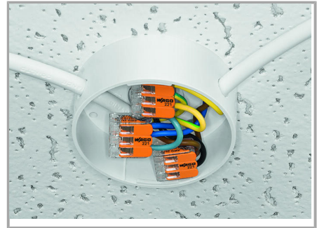
Lighting distribution in ceiling canopy
