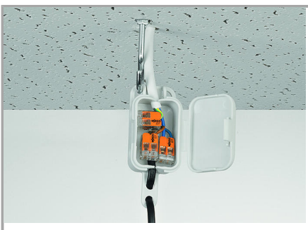
Pendant light connection in suspended ceilings
